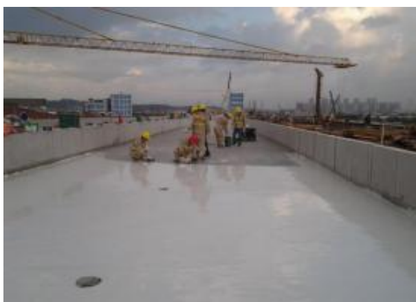
Waterproof layer on the bridge deck of Foshan West Station, Gui-Guang-Nan-Guang Railway
