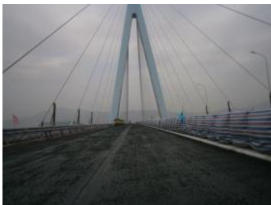
Waterproof bonding layer on the bridge deck of the Xiamen-Zhangzhou Sea-Crossing Bridge
