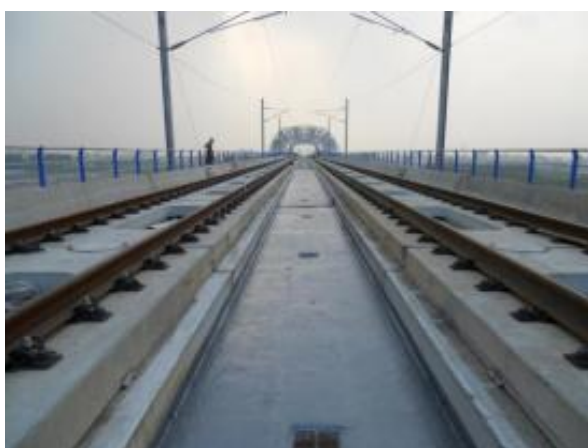
Waterproof layer on the bridge deck of the Shanghai-Nanjing Intercity High-Speed Railway
