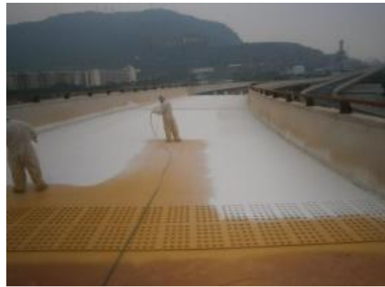
Waterproof layer on the overpass bridge of the Shekou Port Passage, Guangzhou-Shenzhen Coastal Expressway
