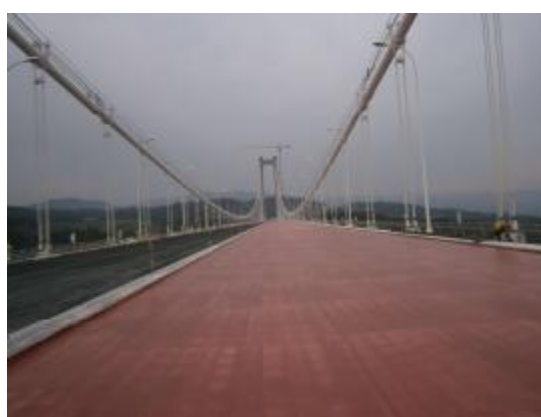
Waterproof bonding layer on the bridge deck of the Tengchong Longjiang Bridge, Yunnan Province
