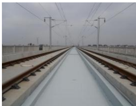
Waterproof layer on the bridge deck of the Guangzhou-Zhuhai Intercity Railway Dongsheng Bridge
