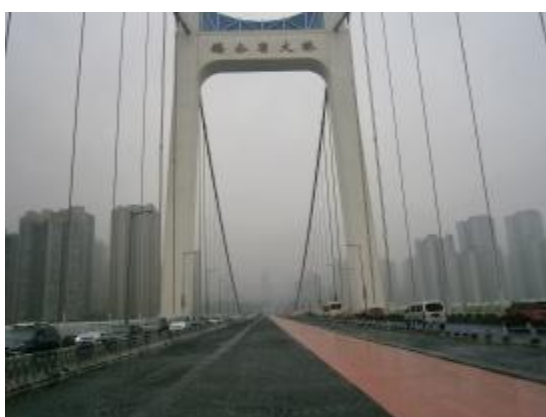
Waterproof bonding layer on the bridge deck of the Chongqing Egongyan Yangtze River Bridge
