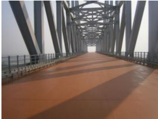
Waterproof and anti-corrosion layer on the bridge deck of the Rongjiang Bridge, Xiamen-Shenzhen High-Speed Railway
