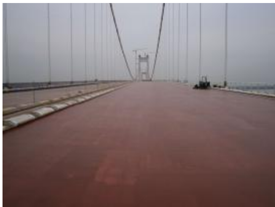
Waterproof bonding layer on the bridge deck of the Ma'anshan Yangtze River Bridge
