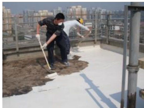
Waterproof layer on the roof of Beijing R&F Residential Area
