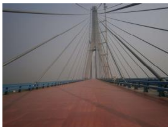
Waterproof bonding layer on the bridge deck of the Tongling Yangtze River Second Bridge (Hefei-Fuzhou High-Speed Railway)
