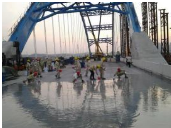
Waterproof layer on the overpass bridge of Foshan West Station, Gui-Guang-Nan-Guang Railway
