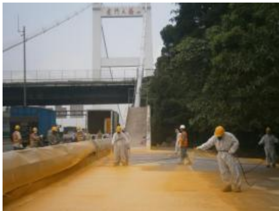
Waterproof protection layer on the main cable anchor of the Humen Bridge
