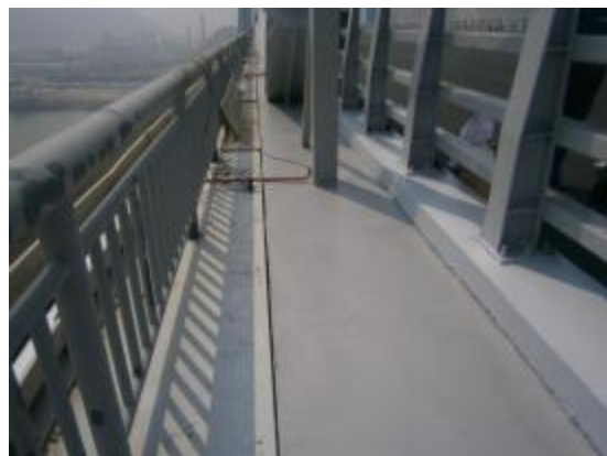
Waterproof layer on the inspection path of the Xiamen-Zhangzhou Sea-Crossing Bridge
